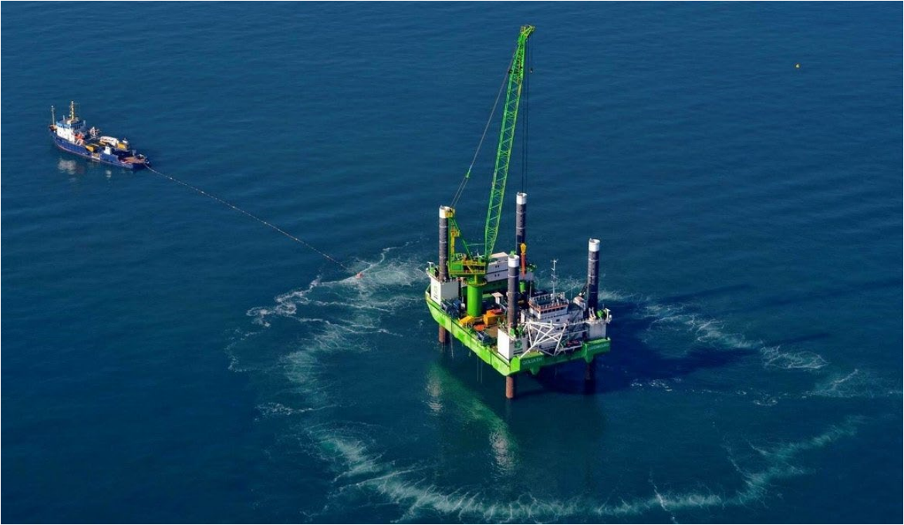
Pile driving operation with bubble curtain. © Trianel/Lang
