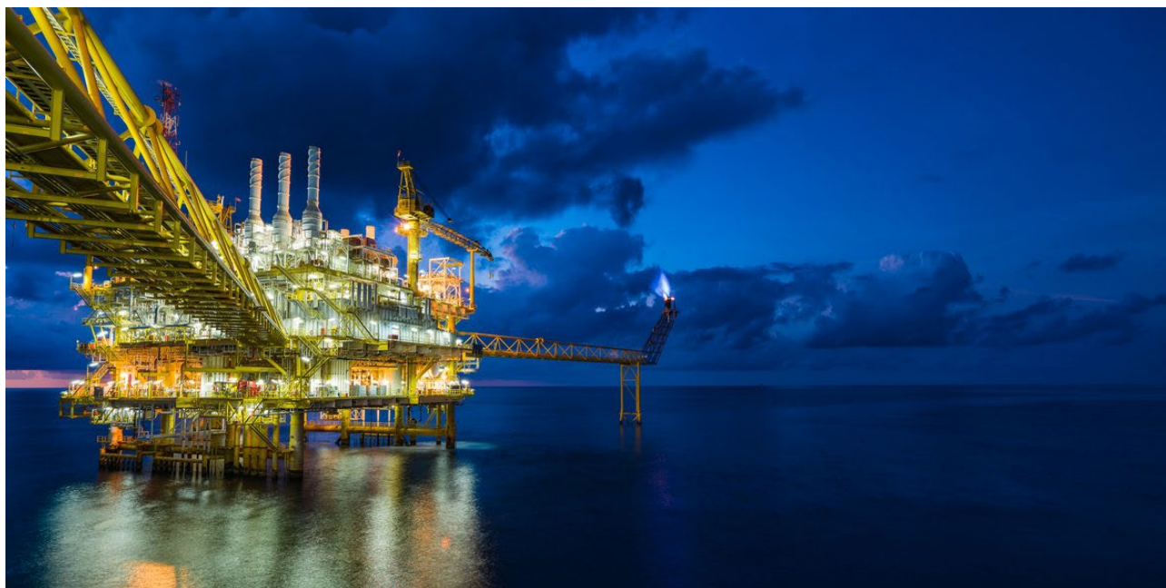
Oil and gas central processing platform. © Shutterstock
