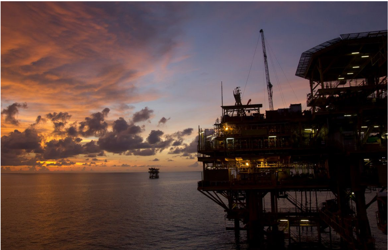
An Oil platform. The Extraction of oil and gas sector identified a decreasing trend in emissions. © Shutterstock
